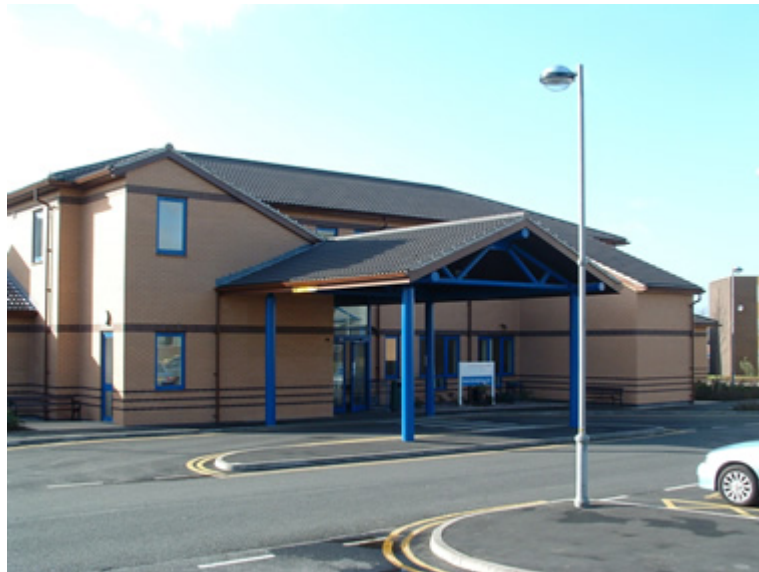
Royal Preston Hospital, Medical Rehabilitation Unit
